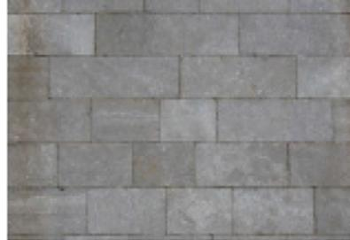
Stone which is cut uniformly on all its exposed surfaces.
